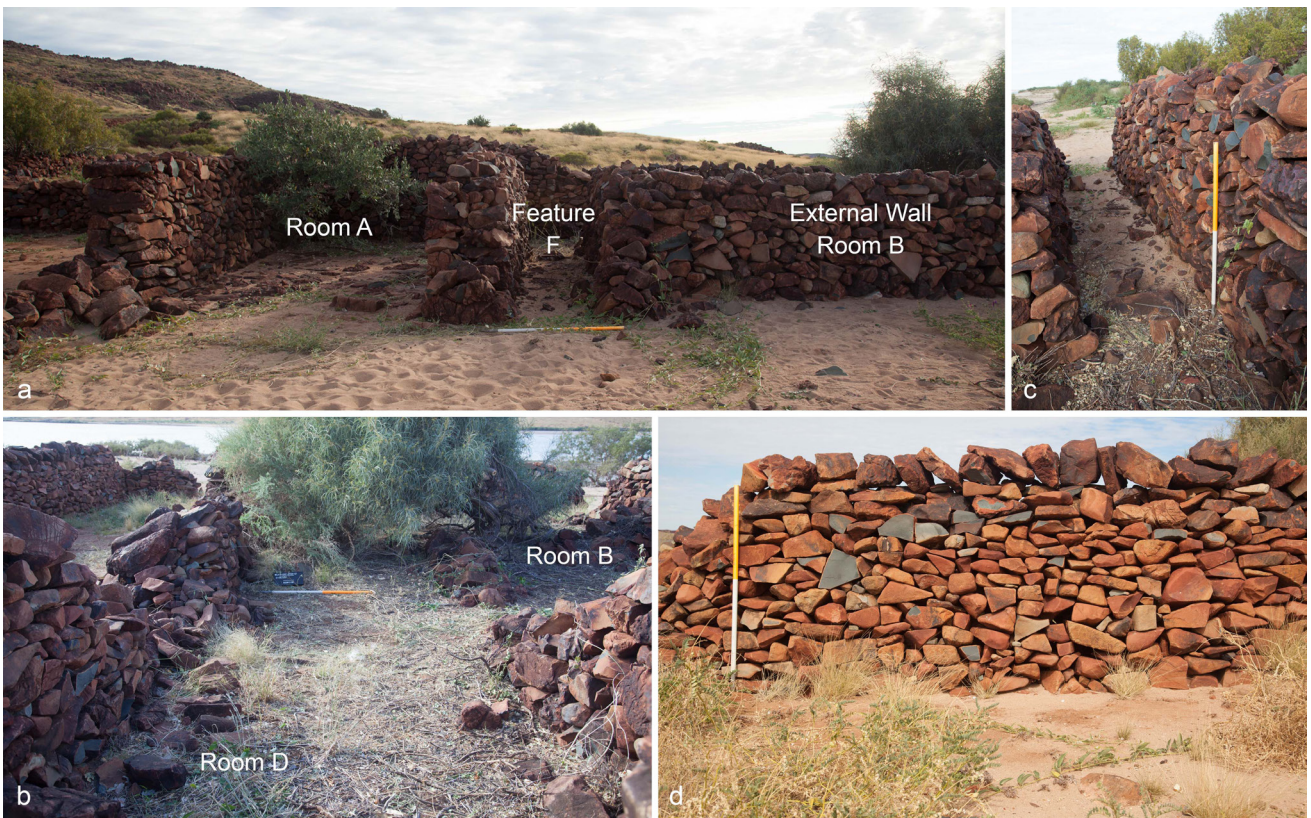
Figure 11.49. Building 7 associated with the sheepyards: (a) view north into Room A and Feature F; (b) Feature F internal, facing south; (c) Room D and entrance into Room B, view east; and (d) high external Wall 3 of Room E.
