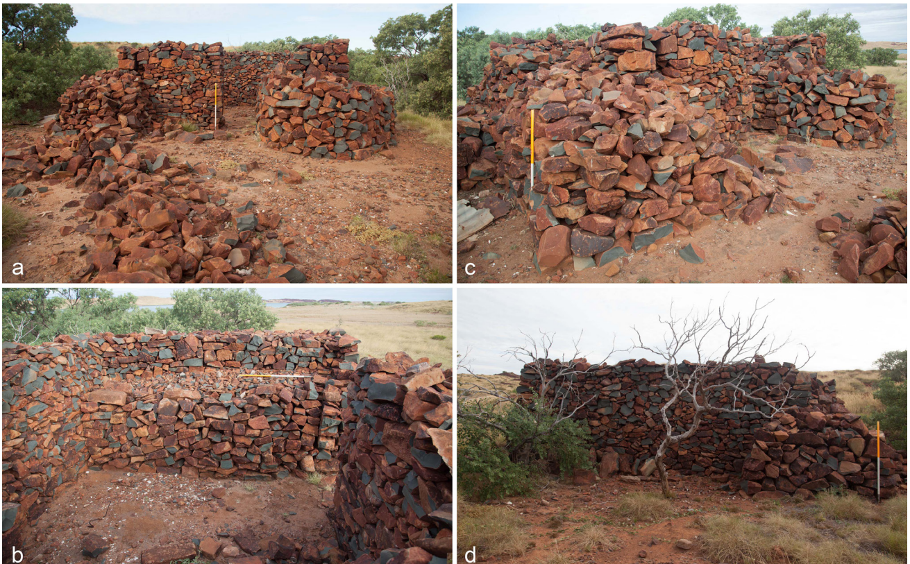
Figure 11.41. (a) View of Building 5 from the west across SWE5; and (b-d) various structural details of Building 5 during the recording.
